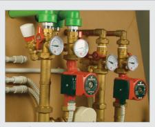
The Giacomini differential pressure valve R147N must be always installed downstream of the pump in between the supply and return pipes, the same versatility allows installation in both horizontal and vertical position respecting the flow direction marked (permanently) on the body itself of the valve.
