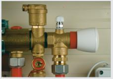
The Giacomini diff erential pressure valve R147N can be installed as an independent component both in the boiler room as well as in the distribution substations (manifold cabinets) and as a subcomponent for preassembled boiler groups Giacomini Series R586 or distribution manifolds R557 for radiant heating system.
